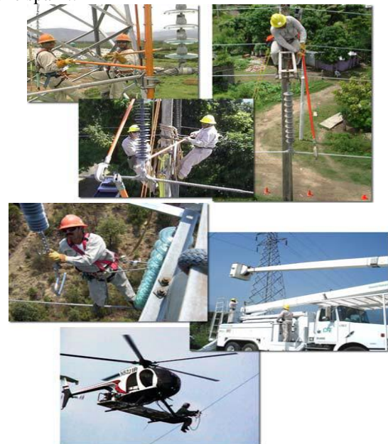
Fig - 8 Some examples of maneuvers for live-line maintenance
