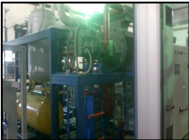
Fig.1. Advance Techno System- Changodar Ahmedabad
