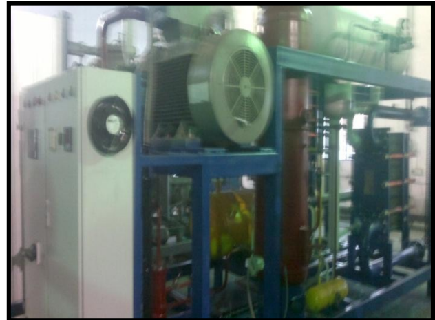
Fig.2. Advance Techno System- Changodar Ahmedabad
