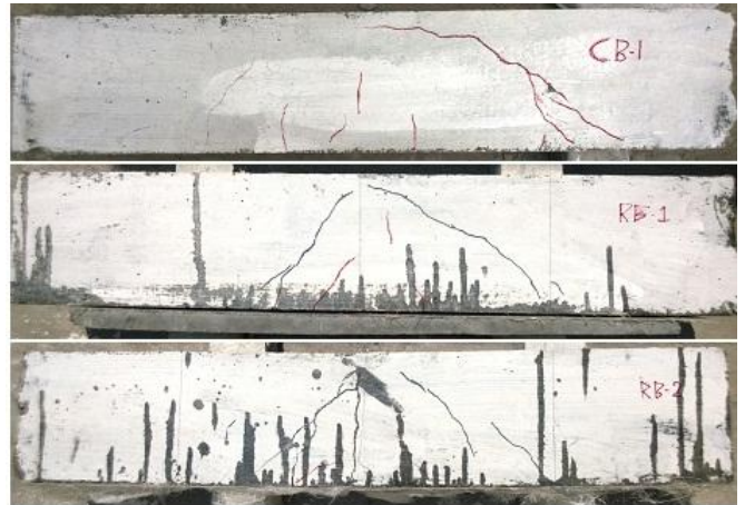
Fig. (7). Crack patterns of the beams after the loading/
