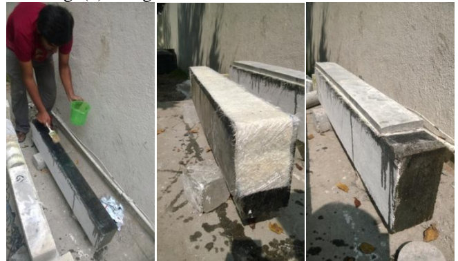
Fig. 5.(1). Application of Epoxy Fig. 5(2). Pasting of Mat Fig. 5(3). Pasting of Laminate
