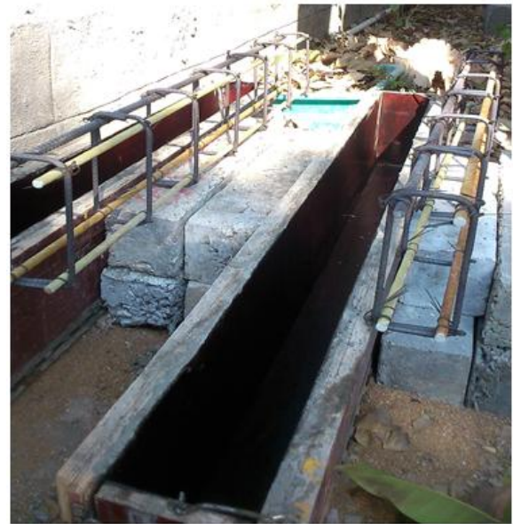
Figure 2: The reinforcement cages before concreting
