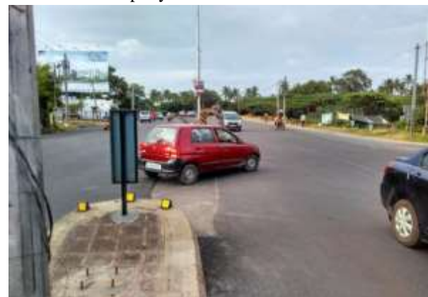
Median opening at Bowenpally stretch
