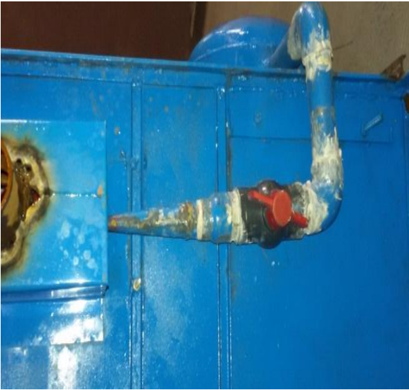
Fig-6 Piping arrangement with nozzle
