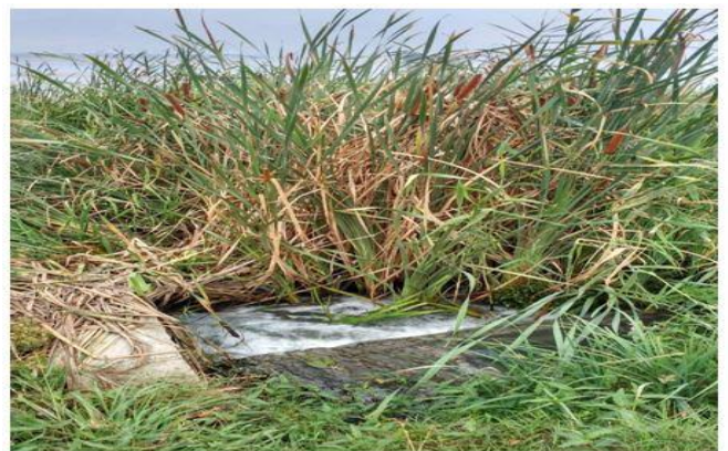
Outfall STP Hazratbal
