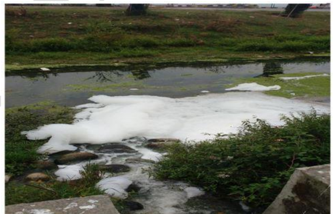
Outfall STP Habak
