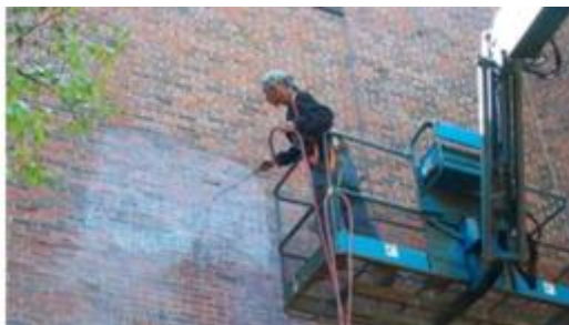
Figure 2: Cleaning of the facade (Restco Corporation, 2013)
