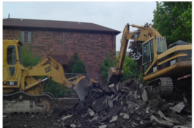
Fig 1: Demolished Asphalt Pavement
