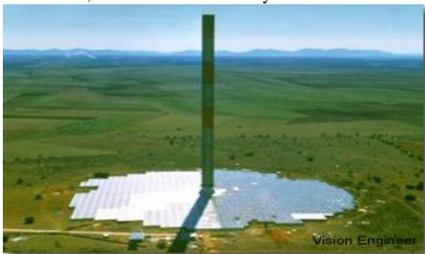
Figure 1: View of solar chimney power plant.
