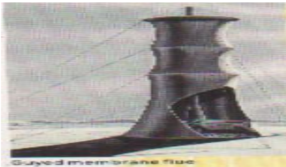
Figure 4: Guyed tube type chimney
