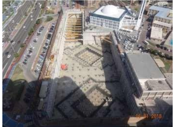
Figure 13 Final View of shoring system in place
