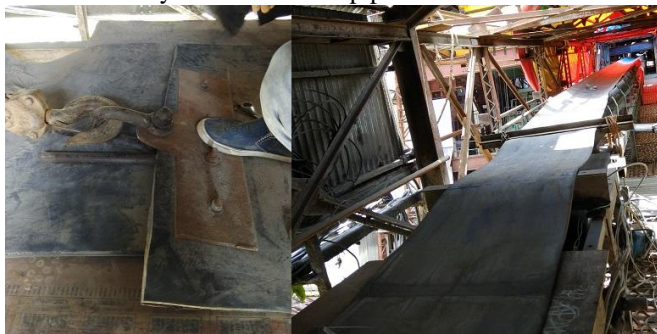
Fig 1: Belt Conveyor (during erection time)
