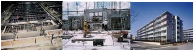
Figure 5 Concrete prefab Source-(Overview of Prefabricated Housing)
