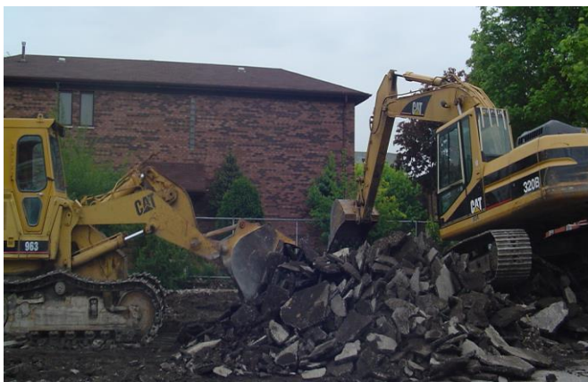
Demolished Asphalt Pavement
