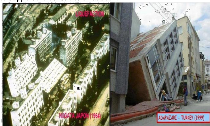
Fig: Liquefaction in Nigata ,Japan (1964) and in Adhapazari Turkey(1999)
