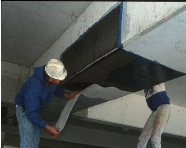
Fig 2- Retrofitting of RCC beam using carbon fibre reinforced sheets. (www.rasonindia.in)
