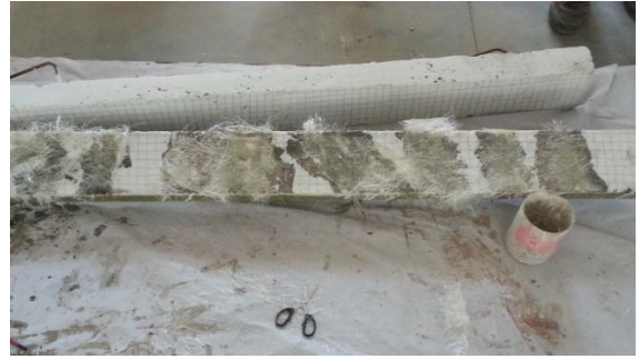
Fig.3 shows that after Partially wrapping of beam by using GFRP
