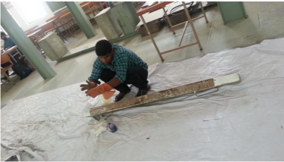
Fig.6 shows that Partial Wrapping of beam by using Bonding plate
