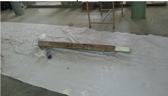
Fig.7 shows after Wrapping of beam by using bonding steel plate
