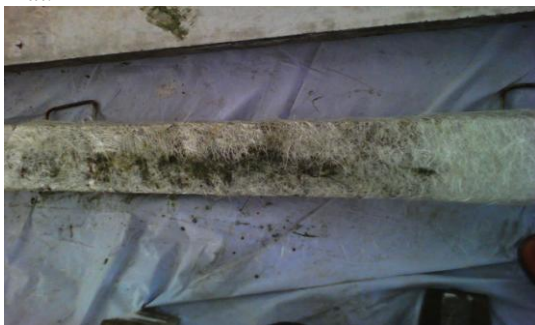
Fig.2 shows that after fully wrapping of beam by using GFRP
