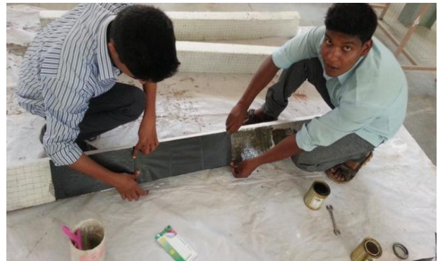
Fig.4 shows that Wrapping of beam by using CFRP
