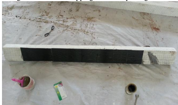
Fig.5 shows that Partial Wrapping of beam by using CFRP
