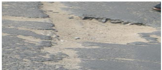
Figure 5. Surface repairs of the canal bridge near Eluru locks
