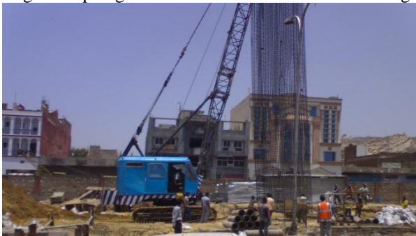
Fig 5. Installation of Reinforcement Frame for Diaphragm Wall
