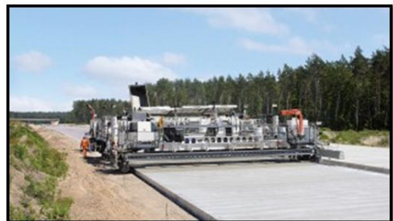
Fig 6 Slipform Paving
