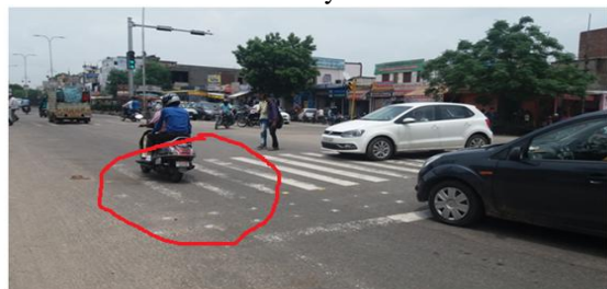
Fig 2 Zebra crossing faded away
