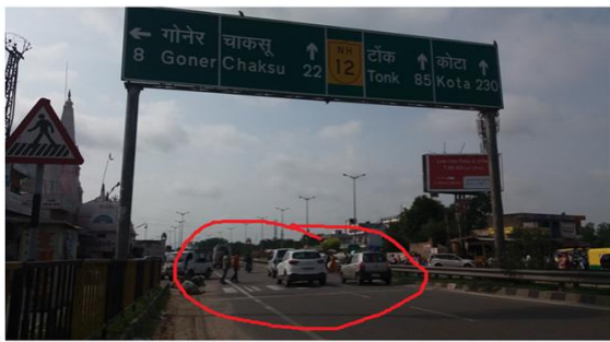
Fig 1 Unsignalised intersection and Zebra crossing faded away
