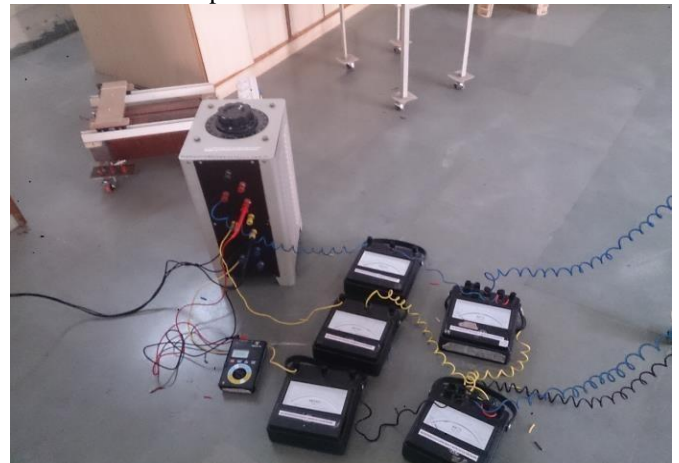
Figure 9: Testing of three phase autotransformer
