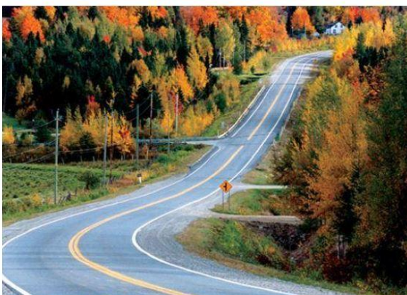
Figure 6.42: Hazardous combination: Hill, intersection, accesses, horizontal curve
