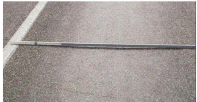
Figure 2.5: Rutting
