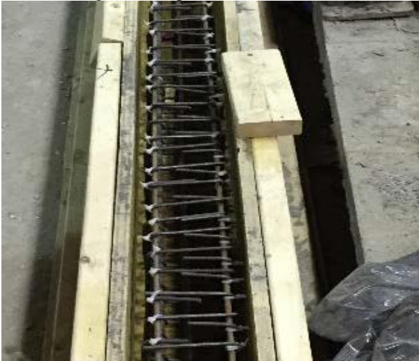
Figure 2: Preparation of R.C Beam
