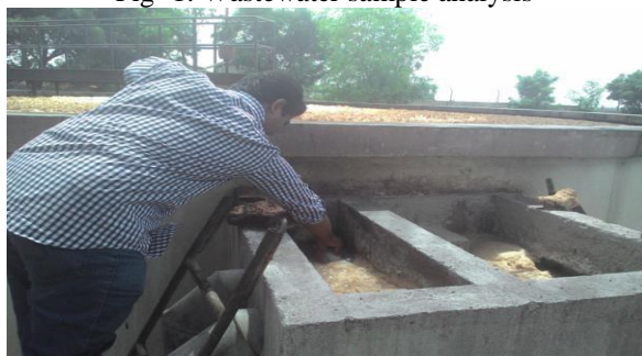
Fig -2: Wastewater sample collection from clarifier
