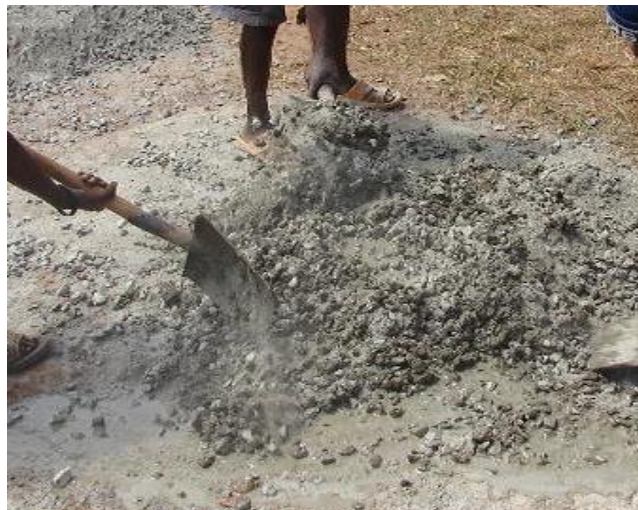
Fig 3.2 Addition of ESP & Copper Slag into Mix
