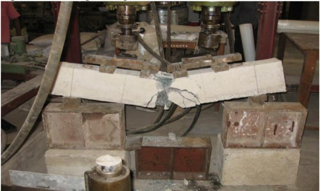
Fig. 5.20 Failure of beam CB1
