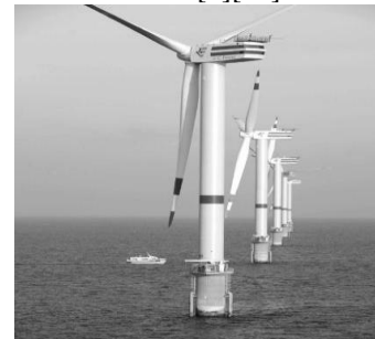
Fig. offshore wind turbine
