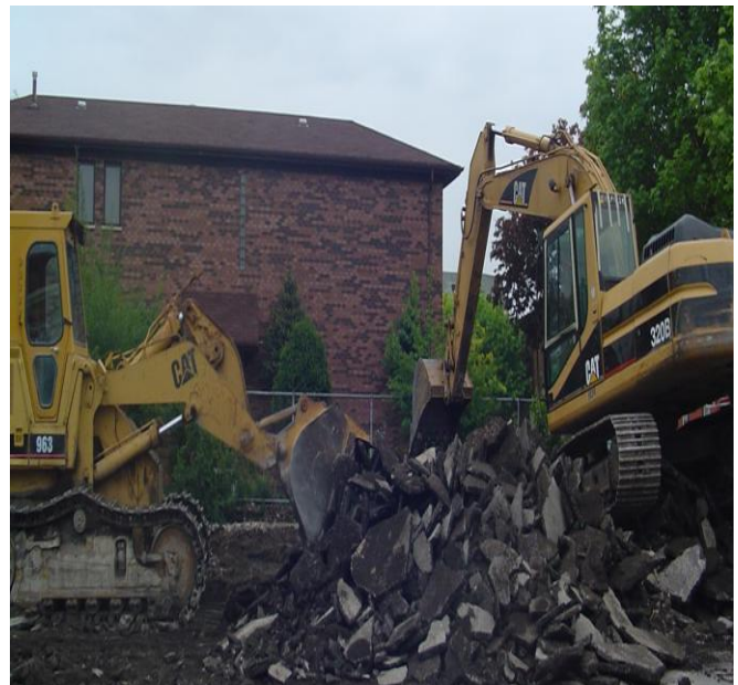
Fig 1: Demolished Asphalt Pavement
