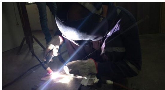
Fig 2.6: Welding of V-butt joint.
