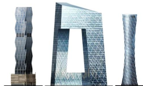
Fig. 1. High Rise Building
