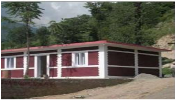
Fig.8. Confined masonry structure defined seismic reinforcement
