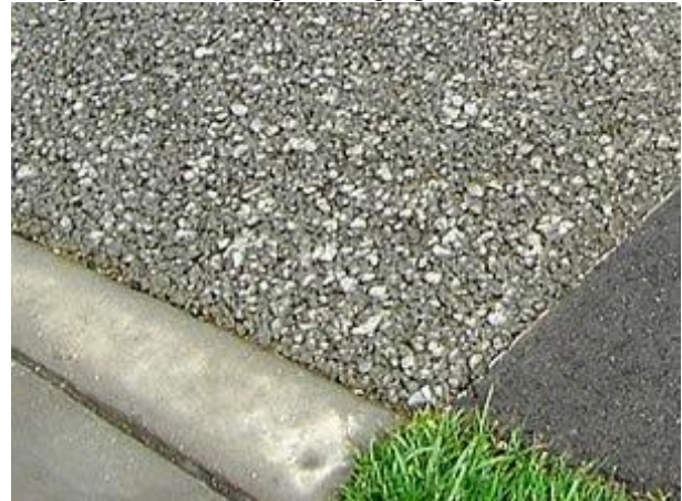
Fig.1 Polish surface of a pervious concrete pavement
