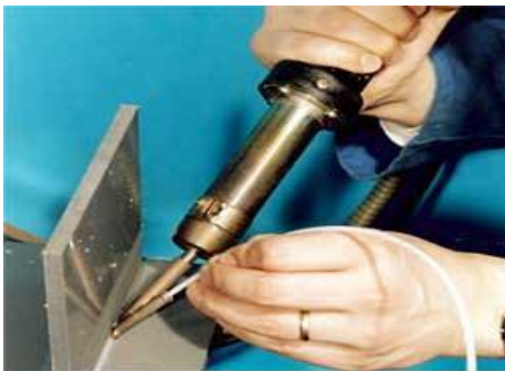
Fig. Hot gas hand welding[8]
