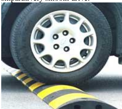
Figure 1: Conventional Speed Breaker
