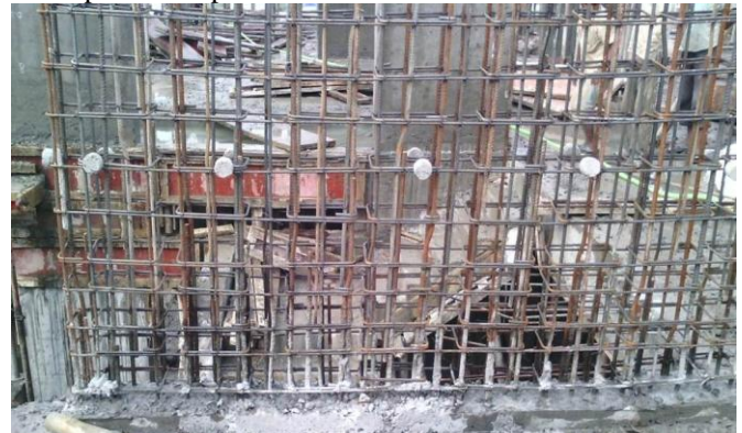
Reinforcement of Shear wall
