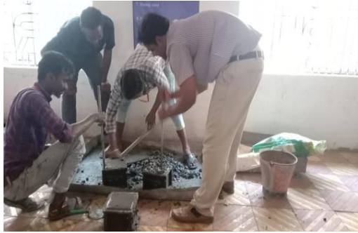
Fig.4 Preparation of cubes
