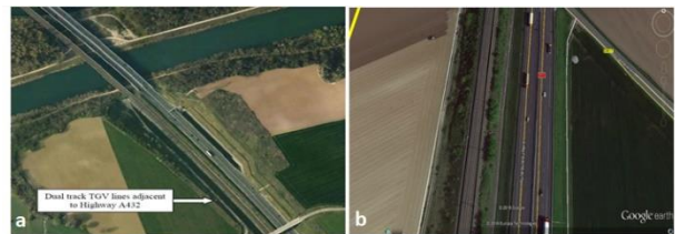
Fig. 13. (a) Two-way TGV lines adjacent to the A432 highway, (b) Parallel high-speed railway with the A1 motorway on the route from Paris to Lille in France
