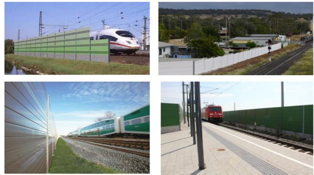
Fig. 8. Use of sound absorbing walls along railway routes
