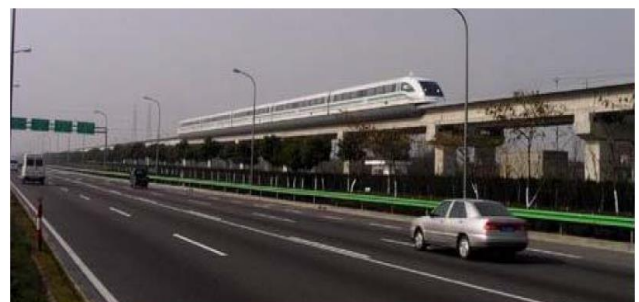
Fig. 10. A side view of a railway and highway parallel project in Shanghai, China
