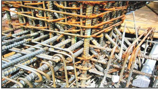
Fig. 1. Congested Reinforcement
