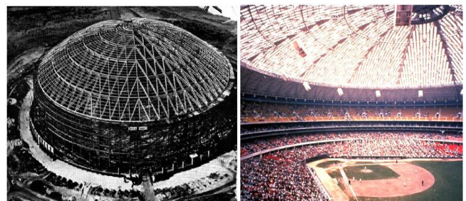
Astrodome (Steel Lamella Dome), Houston/USA
