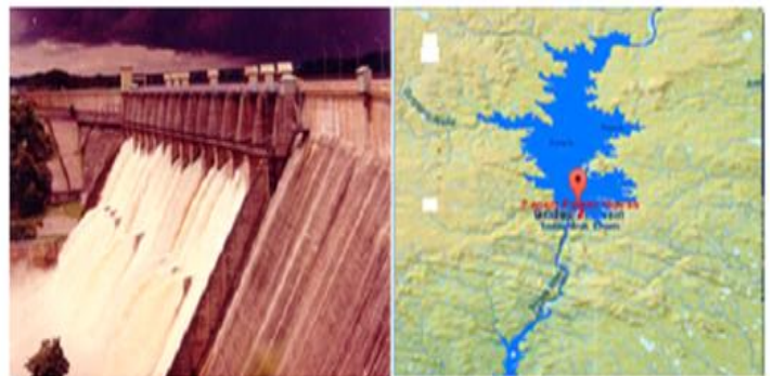
Fig:3.2 Totladoh dam in Fig:3.3 Totladoh dam on Maharashtra Pench river
