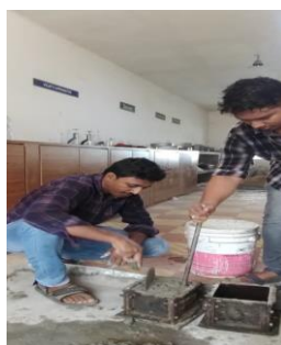
Fig. 4: casting of cubes.
