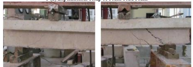
3 (b) Hair line crack started at 110kN
