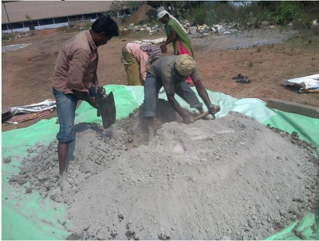
Plate 4.3 Flyash mixing with Expansive Soil
