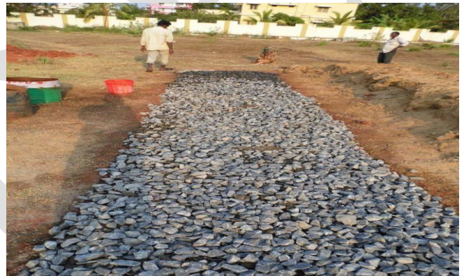
Plate 4.8 Process of laying the Base Course
