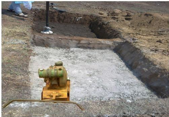
Plate 4.4 Untreated and Treated Subgrade
