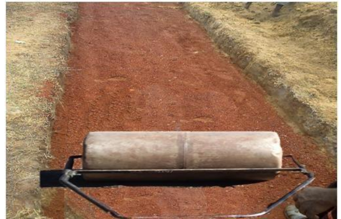
Plate 4.6 Subbase compaction with Hand Held Roller
