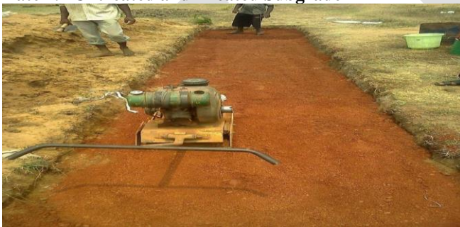
Plate 4.5 Subbase compaction with Earth Rammer
