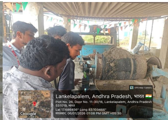
Fig. 3.3 Mixing of Mortar
