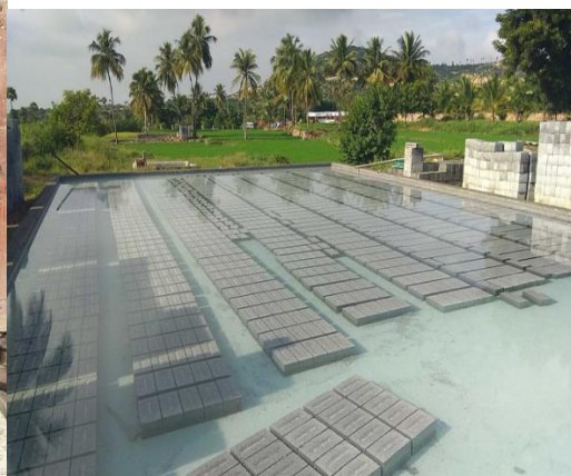
Fig. 3.7 Water curing of FABs
